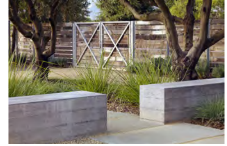
Board form Concrete Seat Walls
