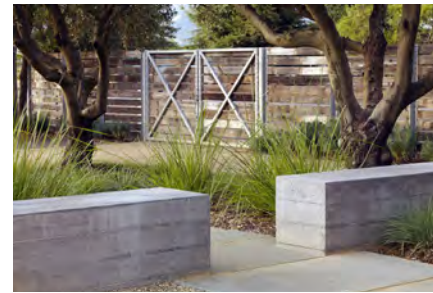
Board form Concrete Seat Walls
