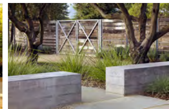
Board form Concrete Seat Walls
