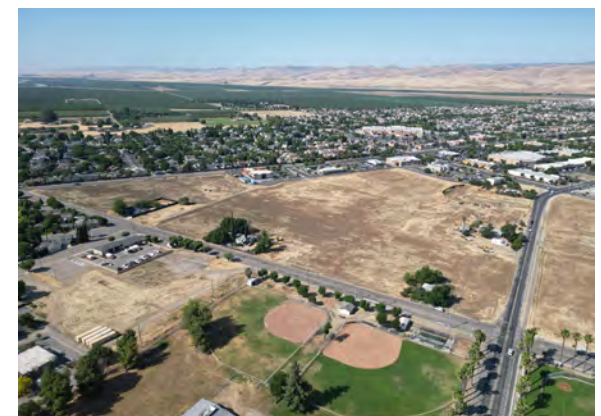
View 4 View of the southern parcel from east looking south west
