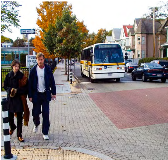
Raised intersection, materiality, traffic calming
