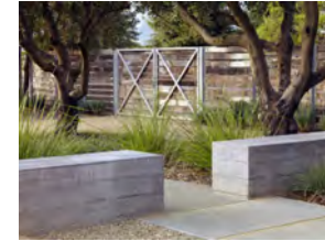
Board form Concrete Seat Walls or Planters
