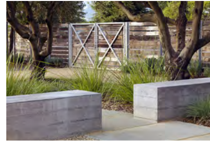
Board Form Concrete Seat Walls
