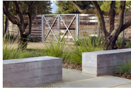
Board form Concrete Seat Walls
